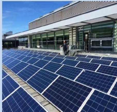
1. Penrhos Depot PV installation – 22.79kW - as part of the construction of the new offices at Penrhos depot, a 22.79kW solar photovoltaic system was installed at the site.
