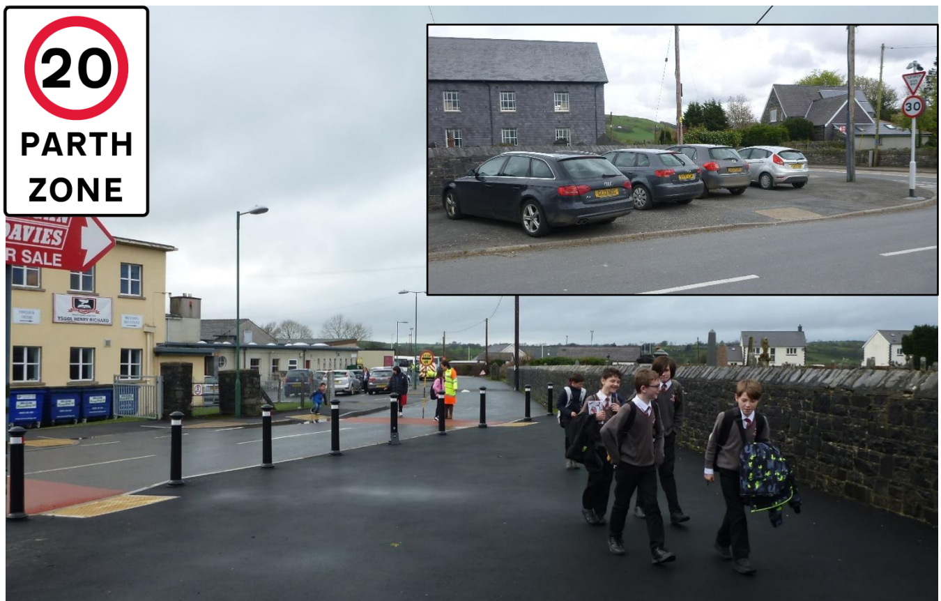
Below: Pre and post scheme photos showing road safety improvements at the school entrance.
