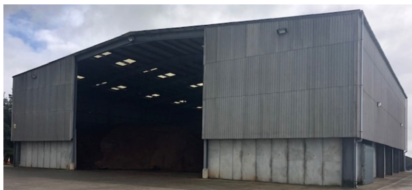
Figure 21 – Salt Barn at Penrhos Depot, Llandysul. Capacity = 6,400 tonnes
