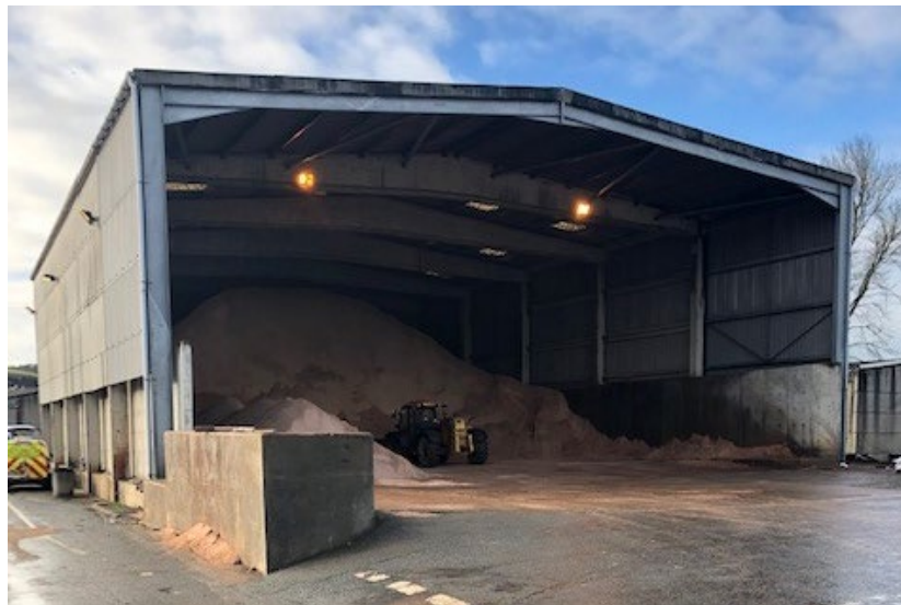
Figure 20 – Salt Barn at Glanyrafon Depot, Aberystwyth. Capacity = 3,400 tonnes.
