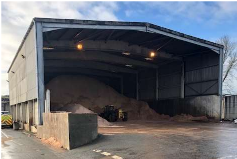
Figure 17 – Salt Barn at Glanyrafon Depot, Aberystwyth. Capacity = 3,400 tonnes.
