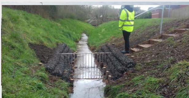
*Through the Small Scale Works Grant 2018/19, Monmouthshire County Council accessed funding to deal with a surface water flooding issue around the Rockfield Estate in Monmouth. Flooding had occurred as a result of blockages to the main trash screen over a culvert.*
