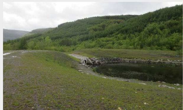
*The project redesigned the existing weir to provide storm water attenuation within the upper catchment area during heavy rain, reusing reclaimed materials.*
